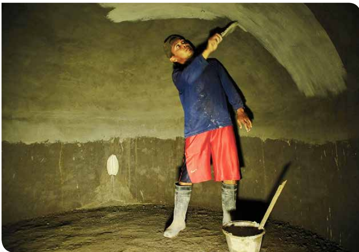
Biogas construction plant in Yogyakarta (photo by Rumah Energi)
